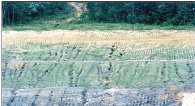
Figure 7.5. Rills and gullies on slopes.
