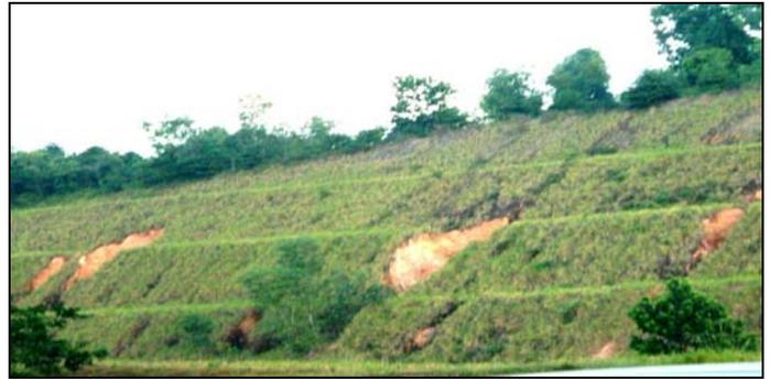
Figure 7.6. Localised slip failures and erosions on slopes.
