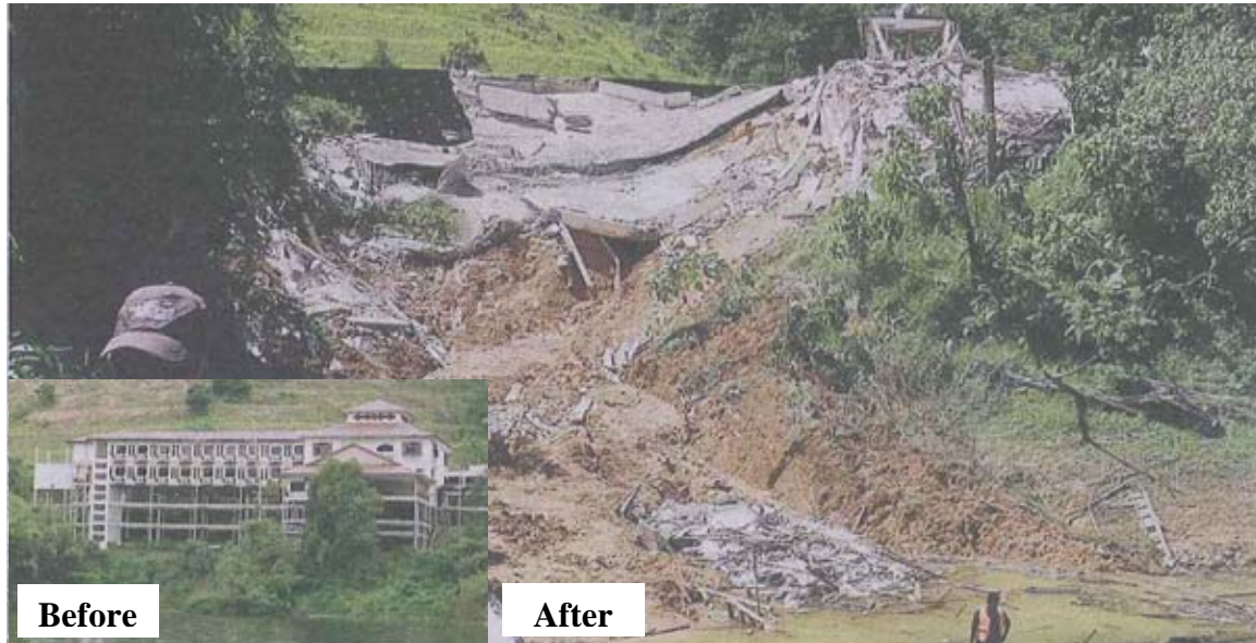
Figure 8: Collapse of Tourism Complex in Pulau Banding, 2007 (The Star, 15 Nov 2007)
