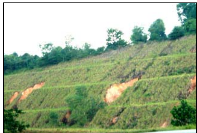
Figure 12: Localized landslips (after Gue & Tan 2004)
