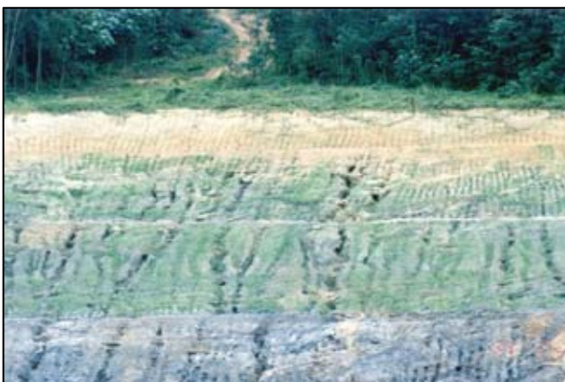
Figure 11: Formation of Rills and Gullies (after Gue & Tan 2004)
