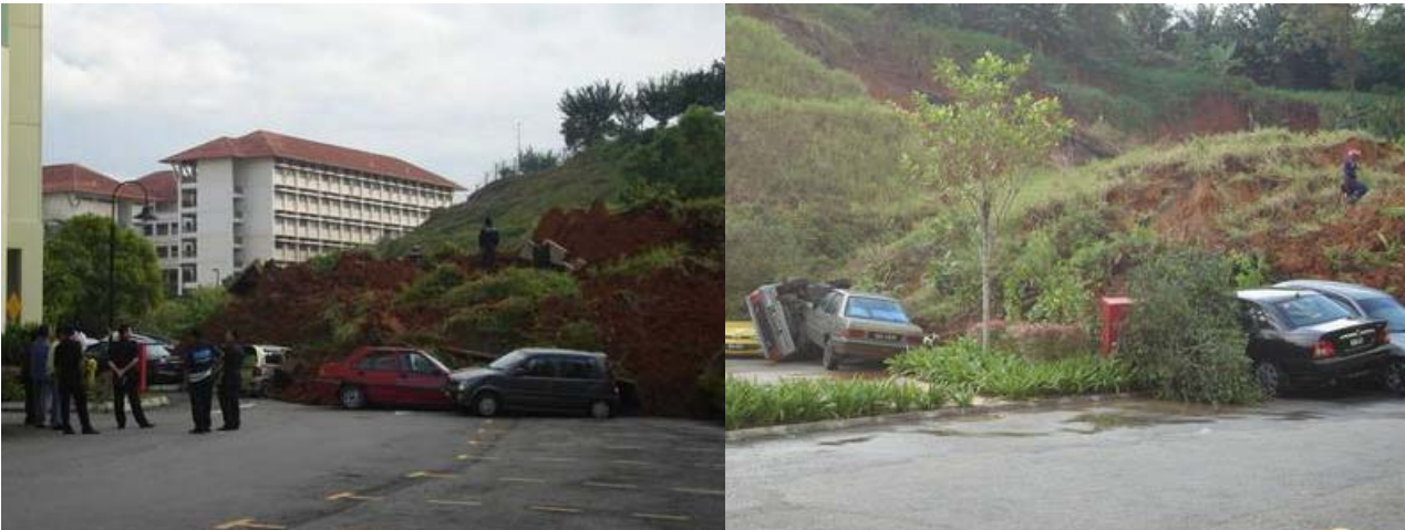
Figure 7: Slope Failure at Precinct 9, Putrajaya, 2007
