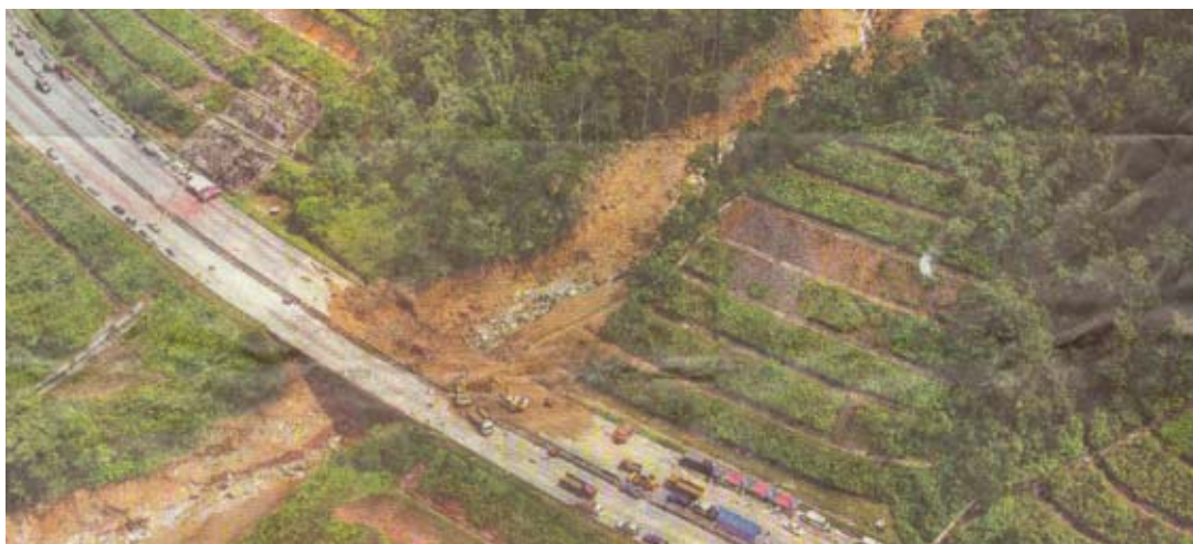
Figure 6: Debris Flow at KM 302 of PLUS Expressway, 2004 (newspaper cutting, Nanyang Siang Pau)
