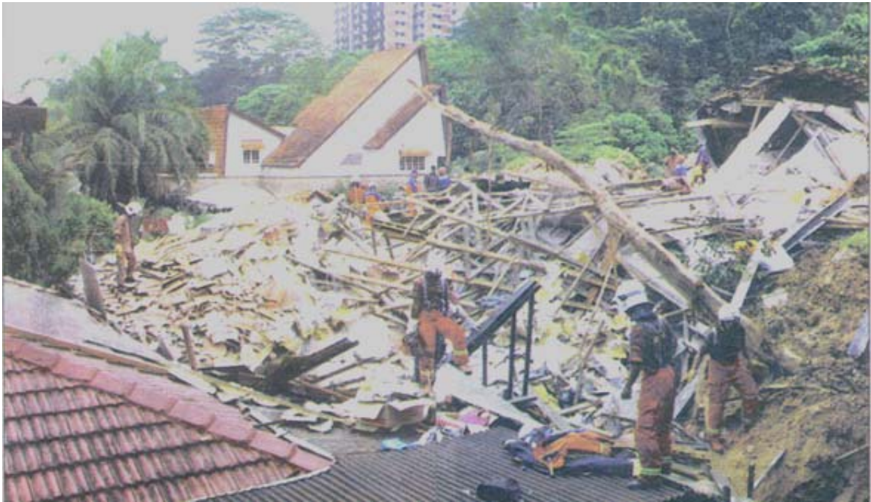
Figure 4: Collapsed Bungalow at Taman Hillview in Ampang, 2003
