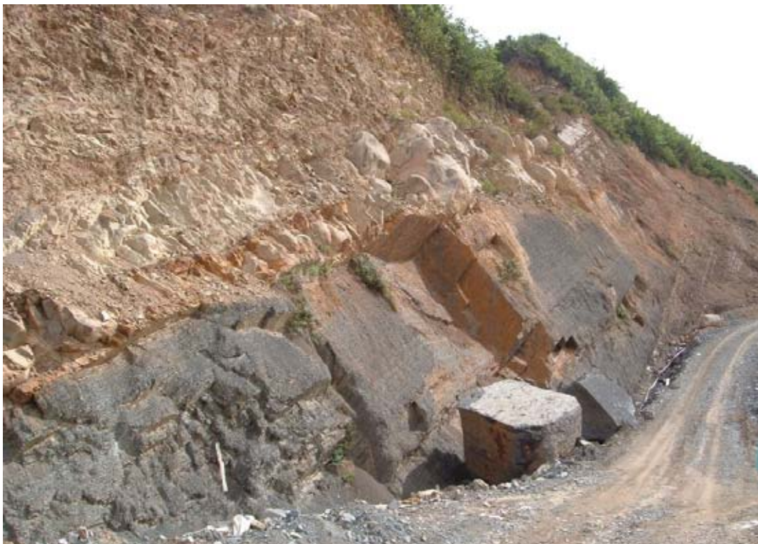
Figure 9: Block Failure of Sedimentary Formation (After Liew S.S. 2005)
