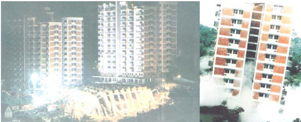
Figure 3: Collapse of Block 1 of Highland Towers Apartments, 1993
