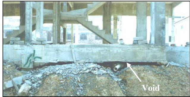
Plate 6 Voids underneath Ground Beam
