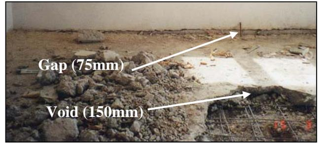
Plate 8 Sagging Ground Floor Slab
