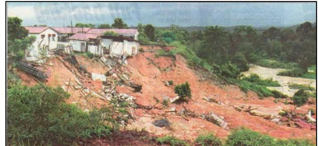
**Plate 14 Failed Slope due to Differential Fill Settlement**
