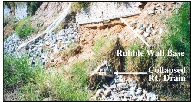
**Plate 10 Collapsed Monsoon Drain**
