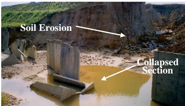
**Plate 13 Erosion Failure of Monsoon Drain**
