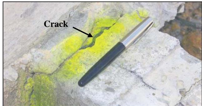
Plate 7 Cracks on Ground Beam
