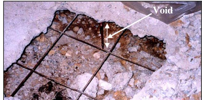
Plate 9 Void underneath the Ground Floor Slab
