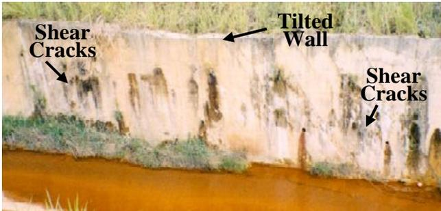
**Plate 12 Shear Cracks on Monsoon Drain**
