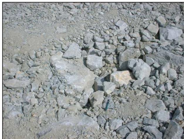
**Plate 5 Poor Compaction around Large Rock**
