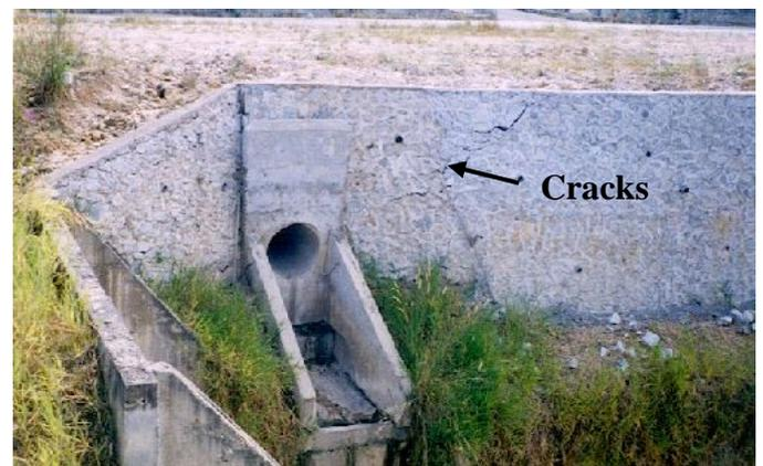
**Plate 11 Shear Cracks on Rubble Wall**
