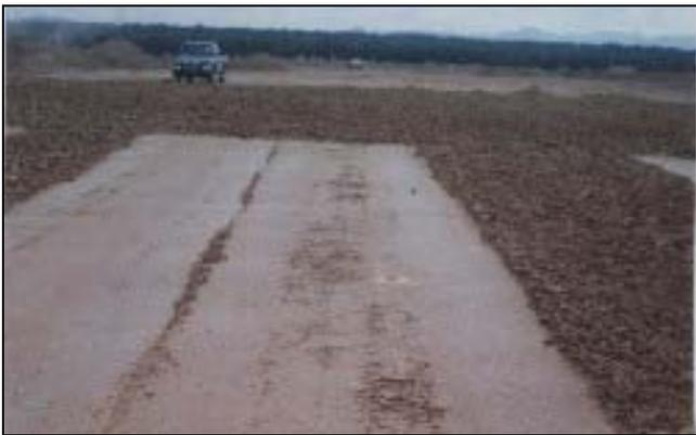
**Plate 2 Smooth Surface of Compacted Soils**
