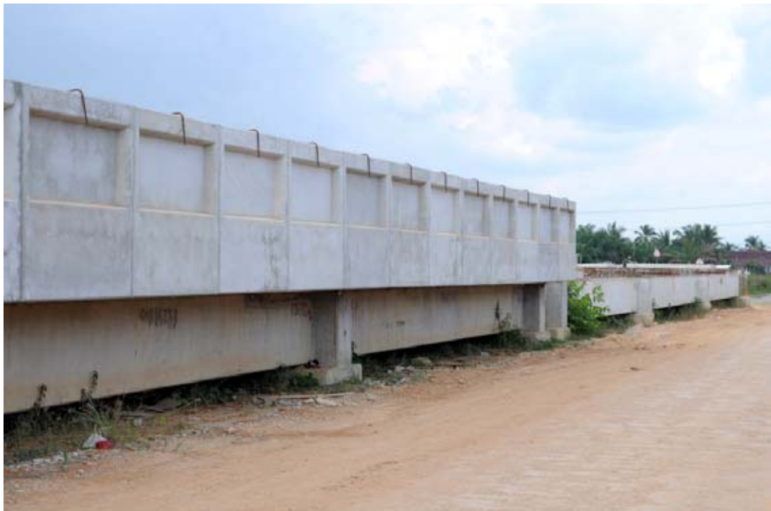
Figure 4: Completed Land Viaduct
