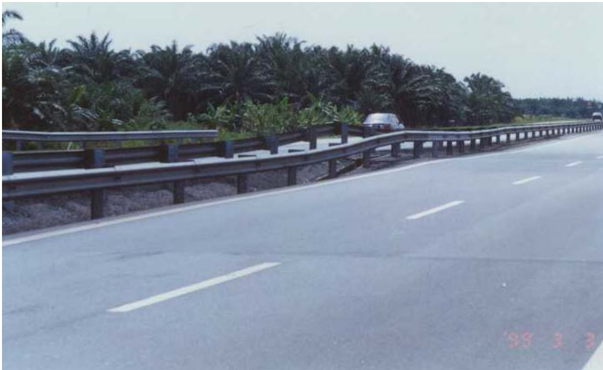
Plate 1: Hump over culvert
